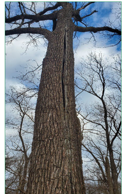
Photograph 2. Example of a stem crack defect.
