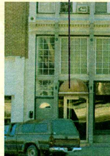
Separated canopies avoid dominating the facade
