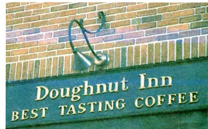
Light shall be directed at the sign from an external, shielded lamp.
