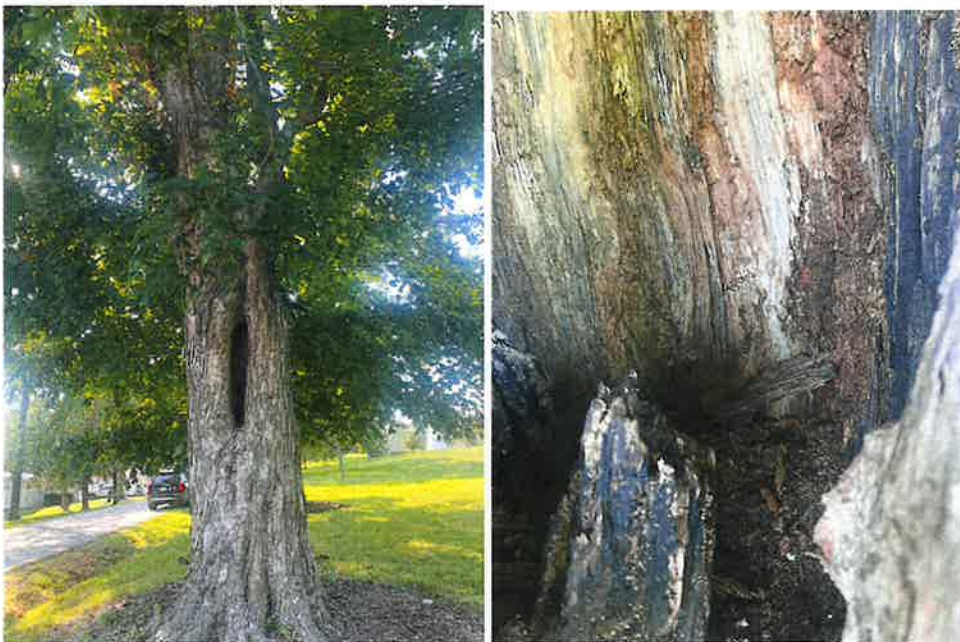
6. Tree needing removal from City Park along Lucky Street, TreeKeeper ID #557 Sugar Maple with severe decay.
